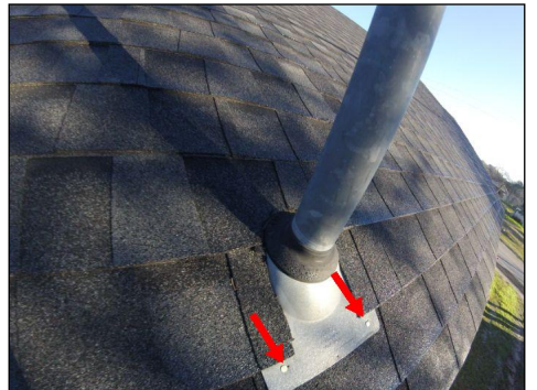
Exposed fasteners at roof flashing
