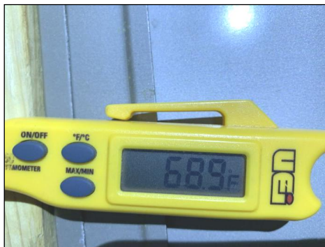
Return Air temperature
