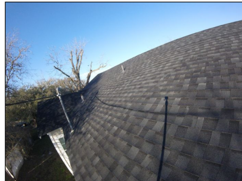
Exposed fasteners at roof flashing
