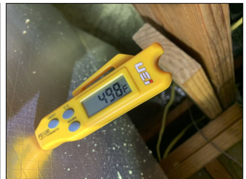
Supply Air temperature
