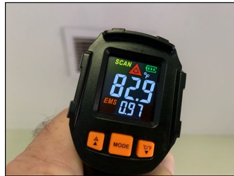
Warmed heating equipment to 82 degrees
