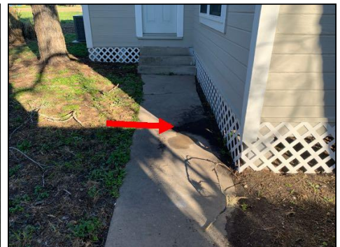
Grade slopes toward the crawlspace at the back of the home
